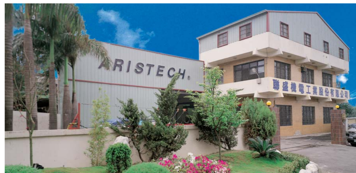
◆ THE FIRST PLANT
